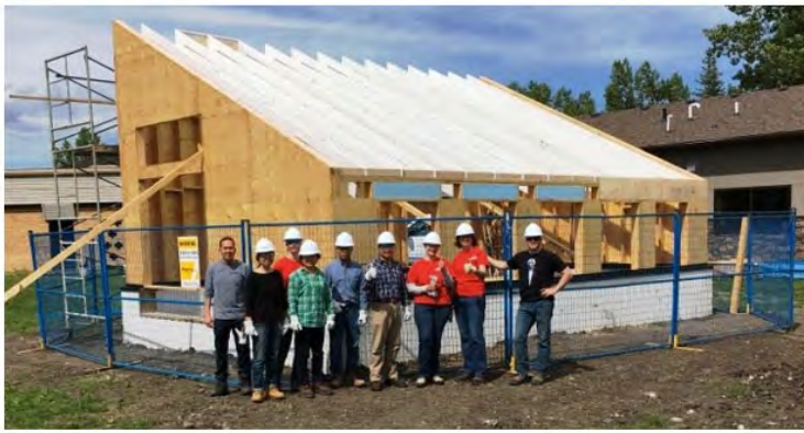
Employees help with the build of the passive solar greenhouse
