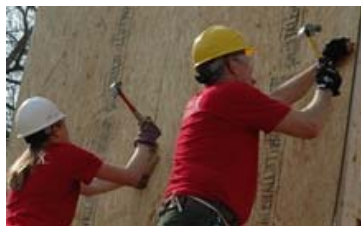
Fluor employees work together to put sheathing on the home.
