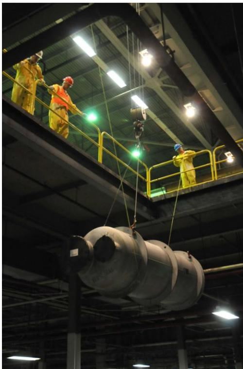
To prepare the site's three massive former enrichment facilities, which are some of the largest buildings in the world, for demolition, workers began sampling and analyzing the contents and then removing the process gas equipment from the X-326 Building. This ongoing process is a key step in total deactivation and equipment removal, allowing D&D of the facility.
